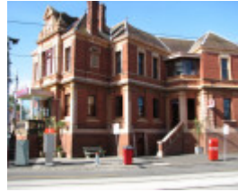
FORMER KEW POST OFFICE SOHE 2008
