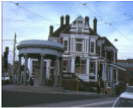
1 former kew post office front view
