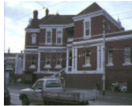
former kew post office cotham road view
