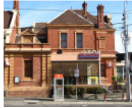
FORMER KEW POST OFFICE SOHE 2008
