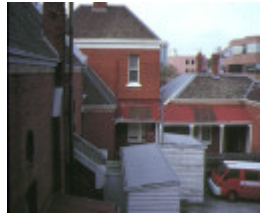
former kew post office rear view
