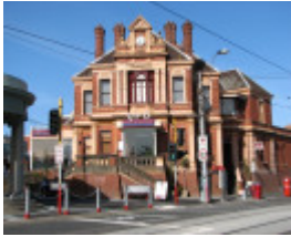
FORMER KEW POST OFFICE SOHE 2008
