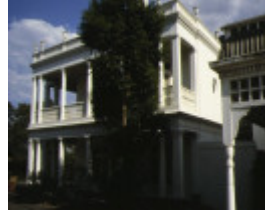
1 studley house kew front view
