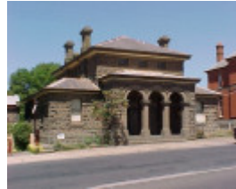
H01471 1 kilmore court house exterior april 2003
