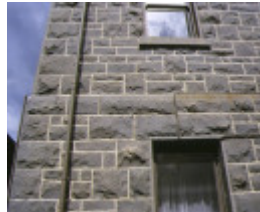
kilmore court house hume highway kilmore blue stone wall detail apr1993
