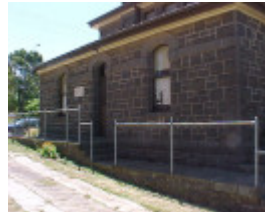
H01471 kilmore court house exterior side april 2003
