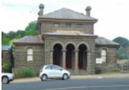
KILMORE COURT HOUSE SOHE 2008
