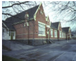
1 primary school no 33 ballarat front elevation aug1984
