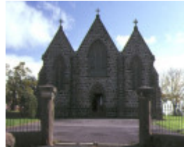
1 st patricks sutherland street kilmore front view may1989
