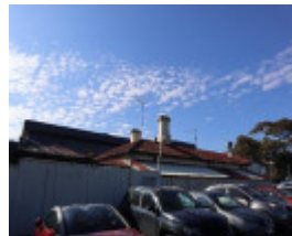
View of the southern elevation
