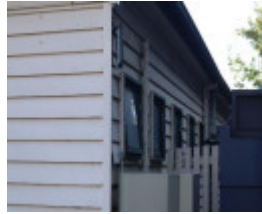
Detail oblique view of the northern face showing new fenestration
