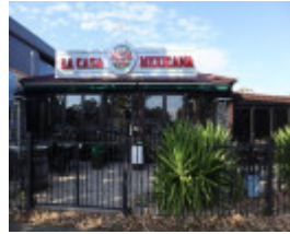
Front view of the west facade from Clyde Road
