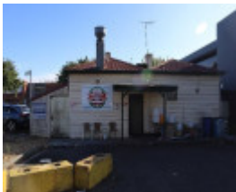
View of the eastern elevation
