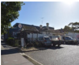
Oblique view of the southern elevation
