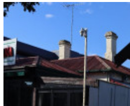
Detail view of the roof and two chimneys looking north east
