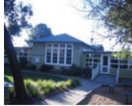
Clyde Primary School - south west view
