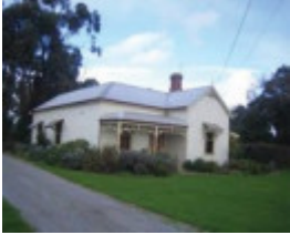
10 Ballarto Road - north east view
