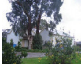
10 Ballarto Road - south east view showing later additions
