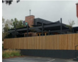
St Agatha s Catholic Church - New addition to north of church
