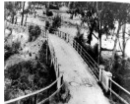
142 - Concrete Arch Bridge Hurstbridge 09 - Old photograph of the bridge - NOTE its approaches and settings - During the 1920s? (ELHPC No.1017) - Shire of Eltham Heritage Study 1992
