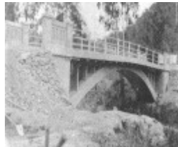
142 - Concrete Arch Bridge Hurstbridge 10 - Old photograph of the bridge - NOTE its approaches and settings - End of construction? (ELHPC No.1055/1061) - Shire of Eltham Heritage Study 1992
