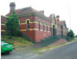
KORUMBURRA RAILWAY STATION COMPLEX SOHE 2008
