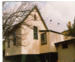
Panton Hill Primary School and Memorial Bell Colour 2 - Shire of Eltham Heritage Study 1992
