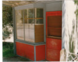
Asbestos Cement Shop Panton Hill Colour 1 - Shire of Eltham Heritage Study 1992
