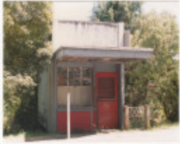
Asbestos Cement Shop Panton Hill Colour 3 - Shire of Eltham Heritage Study 1992
