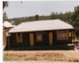
Shop Residence St Andrews Colour 2 - Shire of Eltham Heritage Study 1992
