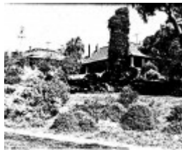
184 - Old Brinkkotter House 32 Lindon Strike Ct 02 - Shire of Eltham Heritage Study 1992
