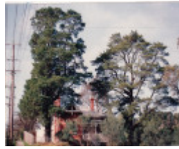
State School 209 Residence Pines 690 Main Rd Colour 4 - Shire of Eltham Heritage Study 1992
