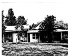
202 - Living Learning Centre 739 Main Rd Eltham 02 - Shire of Eltham Heritage Study 1992
