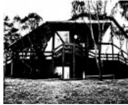
203 - Eltham Community Centre Main Rd Eltham 03 - Shire of Eltham Heritage Study 1992
