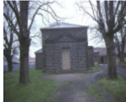
1 kyneton court house hutton street kyneton front elevation sep1984
