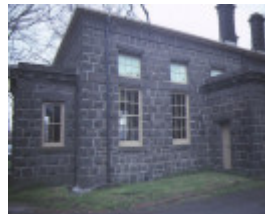
kyneton court house hutton street kyneton side elevation from front sep1984
