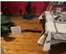
2023. Subfloor bank vault locking mechanism in dining room of the first floor, connects to the bank vault below.
