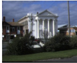
1 former baptist church ballarat front view
