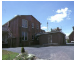
kyneton district hospital simpson street rear view
