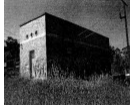
Wattle Glen railway 50hz electricity substation
