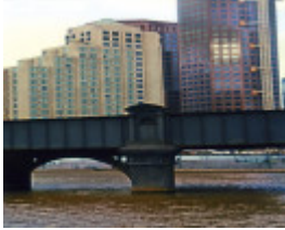
B5620 Sandridge Rail Bridge
