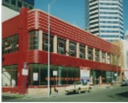
B6256 Former Commonwealth Motors
