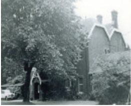
B3137 Vicarage St Peter's Anglican Church
