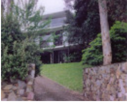
B6035 Delbridge House
