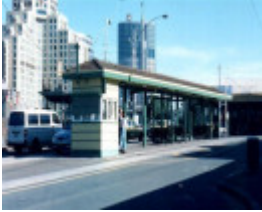
B0435 Batman Avenue Tram Shelter.jpg
