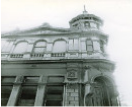
B3404 Former Kensington Property Exchange
