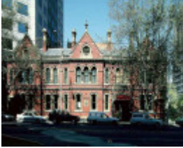
B2477 Former Police Station & Old Police Cells
