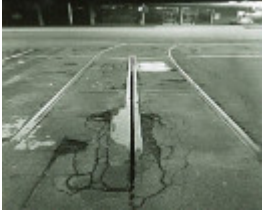
B5088 Cable Tram Tracks
