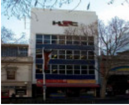
B6348 Barnett's Building
