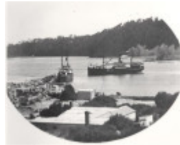
New Works, Lakes Entrance
