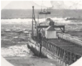
New Works, Lakes Entrance
