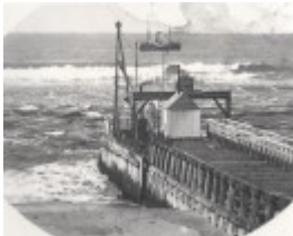
New Works, Lakes Entrance
