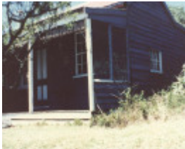
New Works cottage
