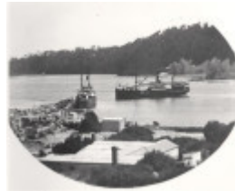
New Works, Lakes Entrance
