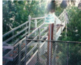
B6321 Middle Brighton Footbridge
