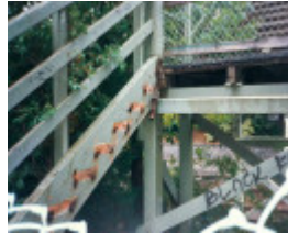
B6321 Middle Brighton Footbridge
