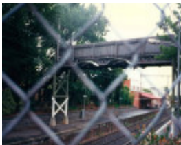
B6321 Middle Brighton Footbridge
