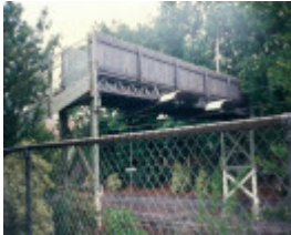
B6321 Middle Brighton Footbridge
