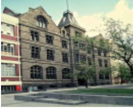
B4621 RMIT Building No 4
