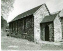
B4820 Former St John the Less Church
