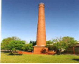
B6871 Boiler House Chimney
