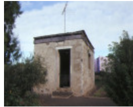
elcho homestead elcho road lara outbuilding
