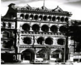
B3058 South Australian Insurance Building
