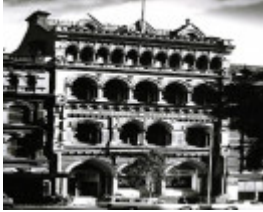
B3058 South Australian Insurance Building
