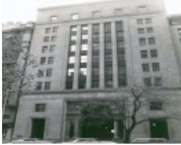
Fmr Commercial Bank of Australia
