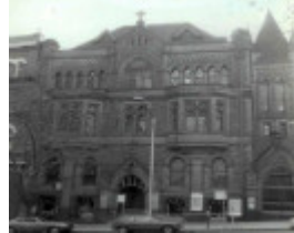
B3900 Fmr Assembly Hall
