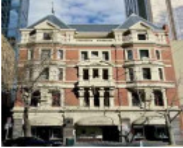
B3927 Austral Building
