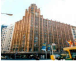
B4080 Manchester Unity Building
