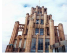
B4080 Manchester Unity Building
