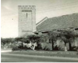
B5908 Former Uniting Church
