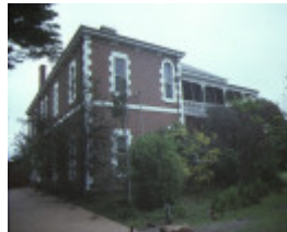
pirra homestead windermere road lara side view sep1984
