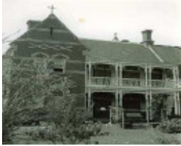
B4381 Presbytery Burwood Road Hawthorn
