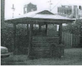
B7041 Tram Shelter
