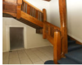
B4908 Canterbury Mansions Entrance Stairway
