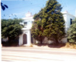
B3811 Former Bridge Hotel
