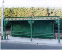
B7039 Cast-iron Tram Shelter
